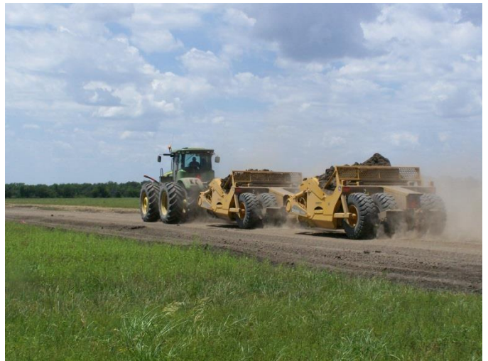
OK USDA-NRCS: 68-7335-1-16 Wetland Reserve Program, Oklahoma Prime Contractor – Contract Value: $800,000.00
