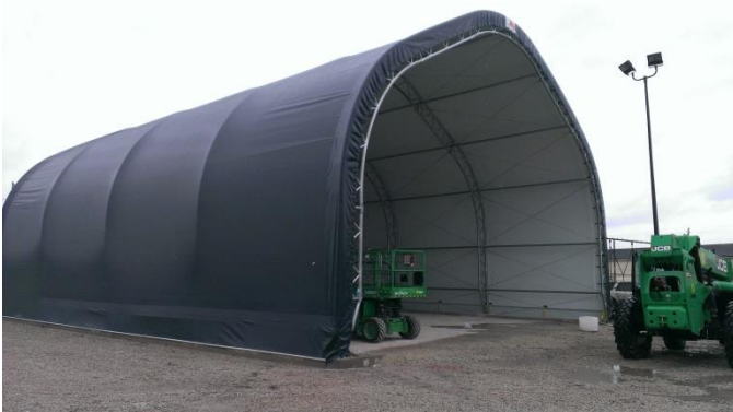
Greater Dayton Regional Transit Authority: GD12-26 Salt Barn, Rammed Aggregate Piers, Dayton Ohio Prime Contractor – Contract Value: $309,214.00
