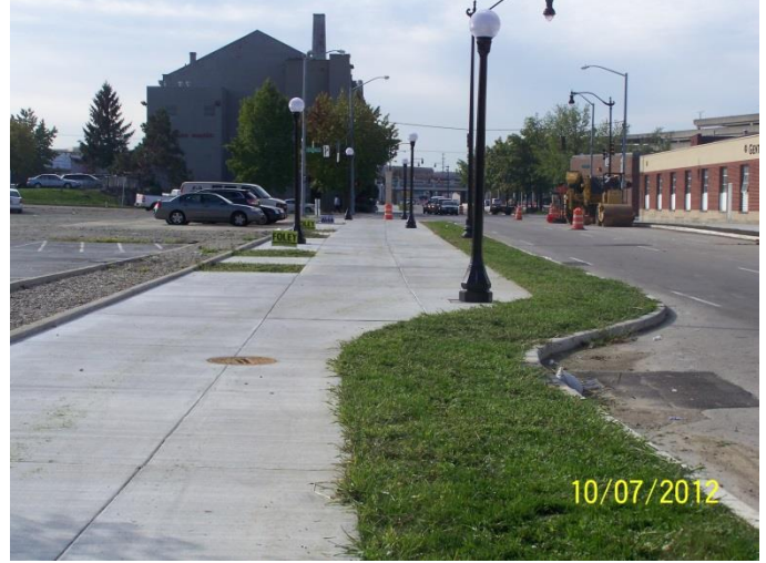
City of Dayton: CT12-0338 Patterson Blvd Canal Pkwy, Dayton, Ohio Prime Contractor – Contract Value: $2,000,000.00
